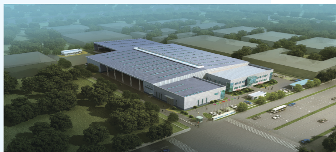
Oil injected screw compressors and refrigerant dryers plant: Pan-Asia, Wuxi
